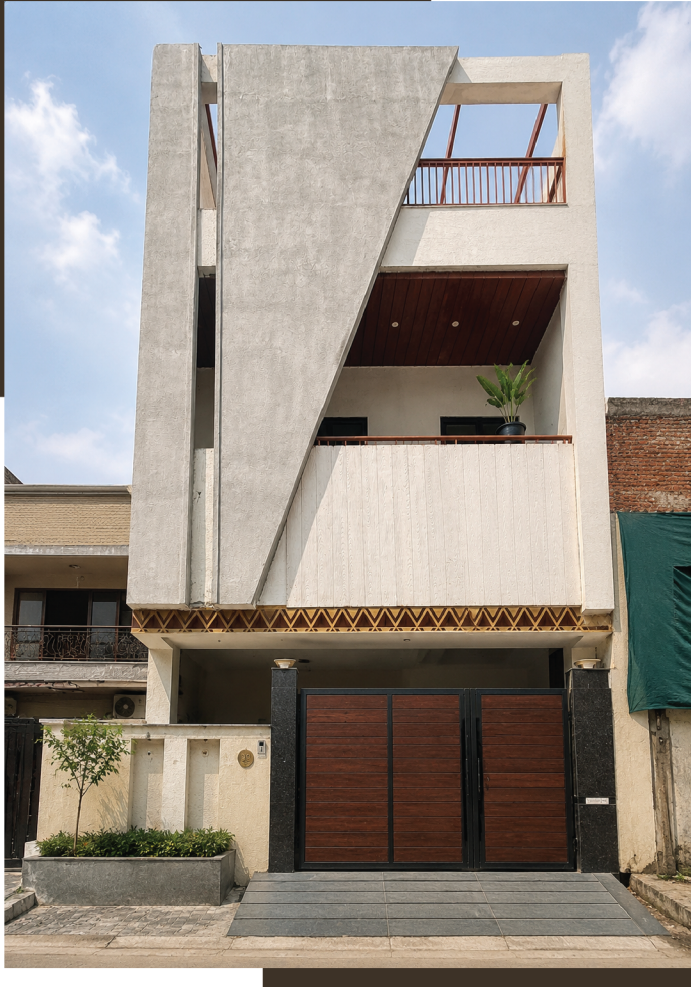
Rough finish to exterior walls for residential site.
